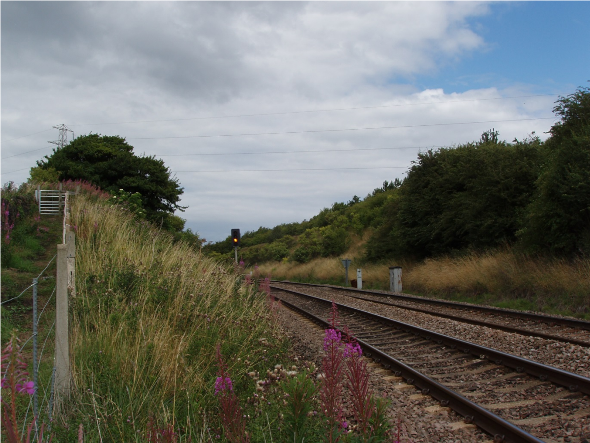
West Side Looking North
